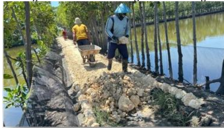
Figure 10. Construction of a Sea Wall via Embankment Filling
