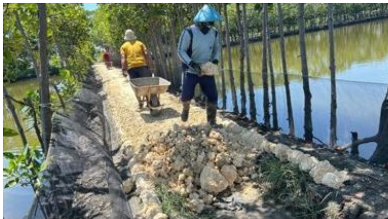
Figure 6. Training on Sea Wall Construction via Embankment Filling
