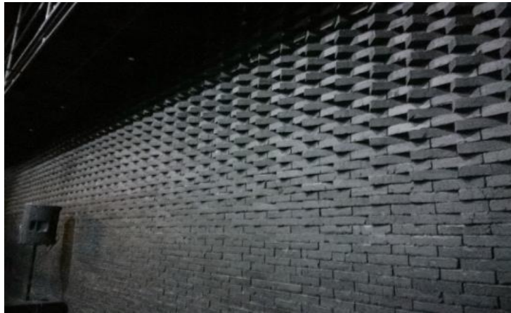
Figure 3. Wall Surface Using Rotating Installed Bricks
