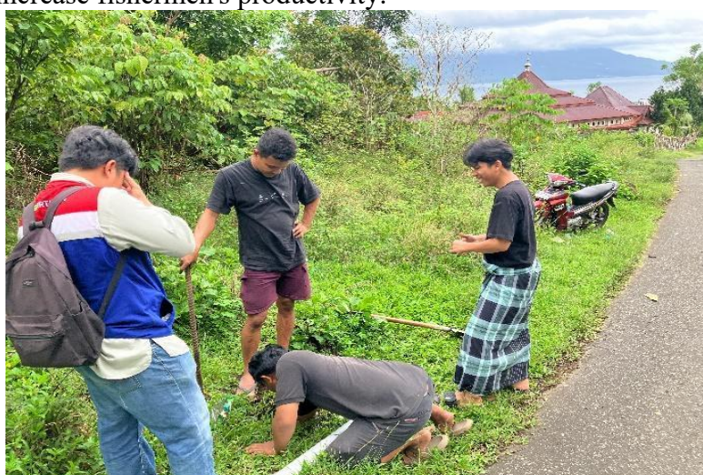
Figure 2. Installation of Solar Panel Lights
