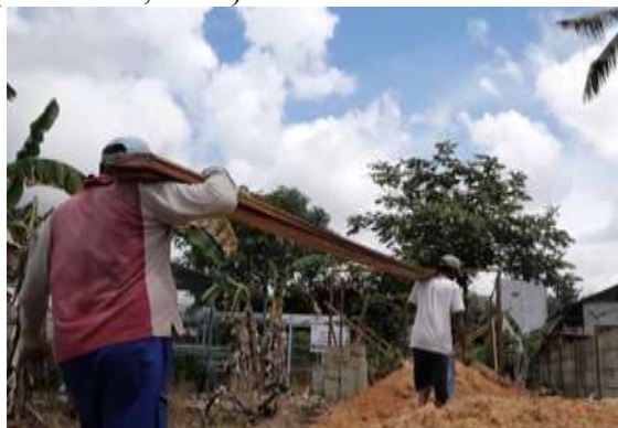
Figure 2. The Process of Building Saung Pandu Warehouse
